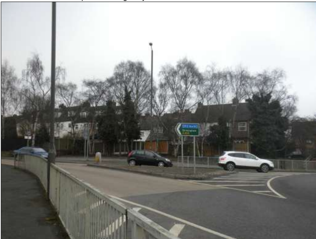
Photo 9 – View of part of the AQMA at Coventry Street island at the junction with Coventry Street, note closeness of receptors to Ring Way.
