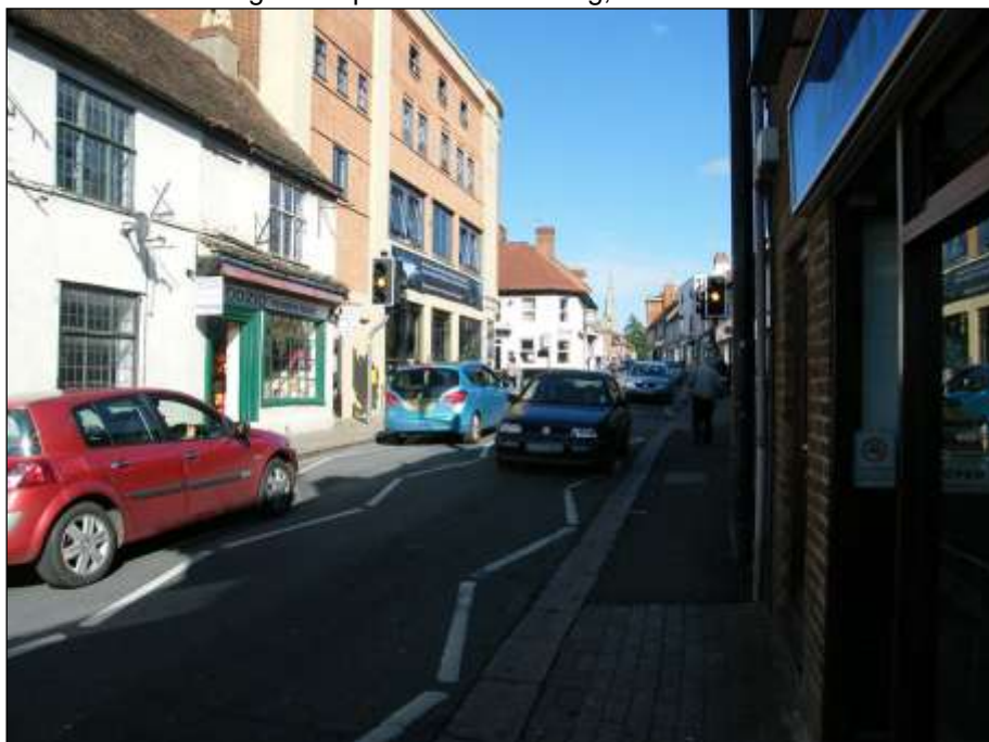
Photo 2: Looking NE to pedestrian crossing, cinema and Burford Road.
